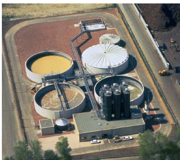
Figure 16.21 (A) EGSB installation for treatment of dairy wastewater in Germany and (B) IC installation for treatment of brewery wastewater in Den Bosch in the Netherlands (photo: Biothane B.V. and Paques B.V. respectively)
