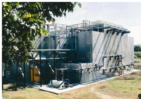
Figure 16.18 UASB installations for treatment of (A) fruit juice factory wastewater in Bregenz, Germany and (B) dairy wastewater in Indonesia (photo: Paques B.V. and Biothane B.V. respectively)
