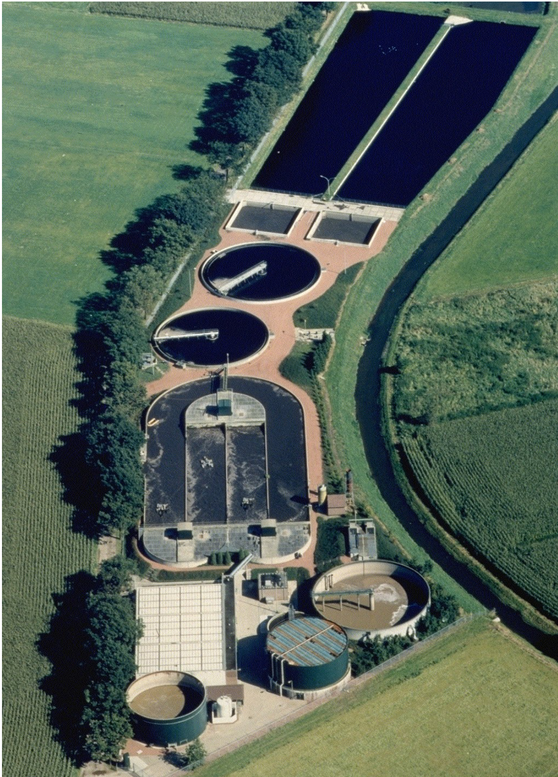
A full-scale application of UASB technology: brewery wastewater treatment plant of Bavaria in Lieshout, the Netherlands. The UASB reactor is placed in front of the Carrousel (photo: J.B. van Lier by courtesy of Bavaria N.V.)
